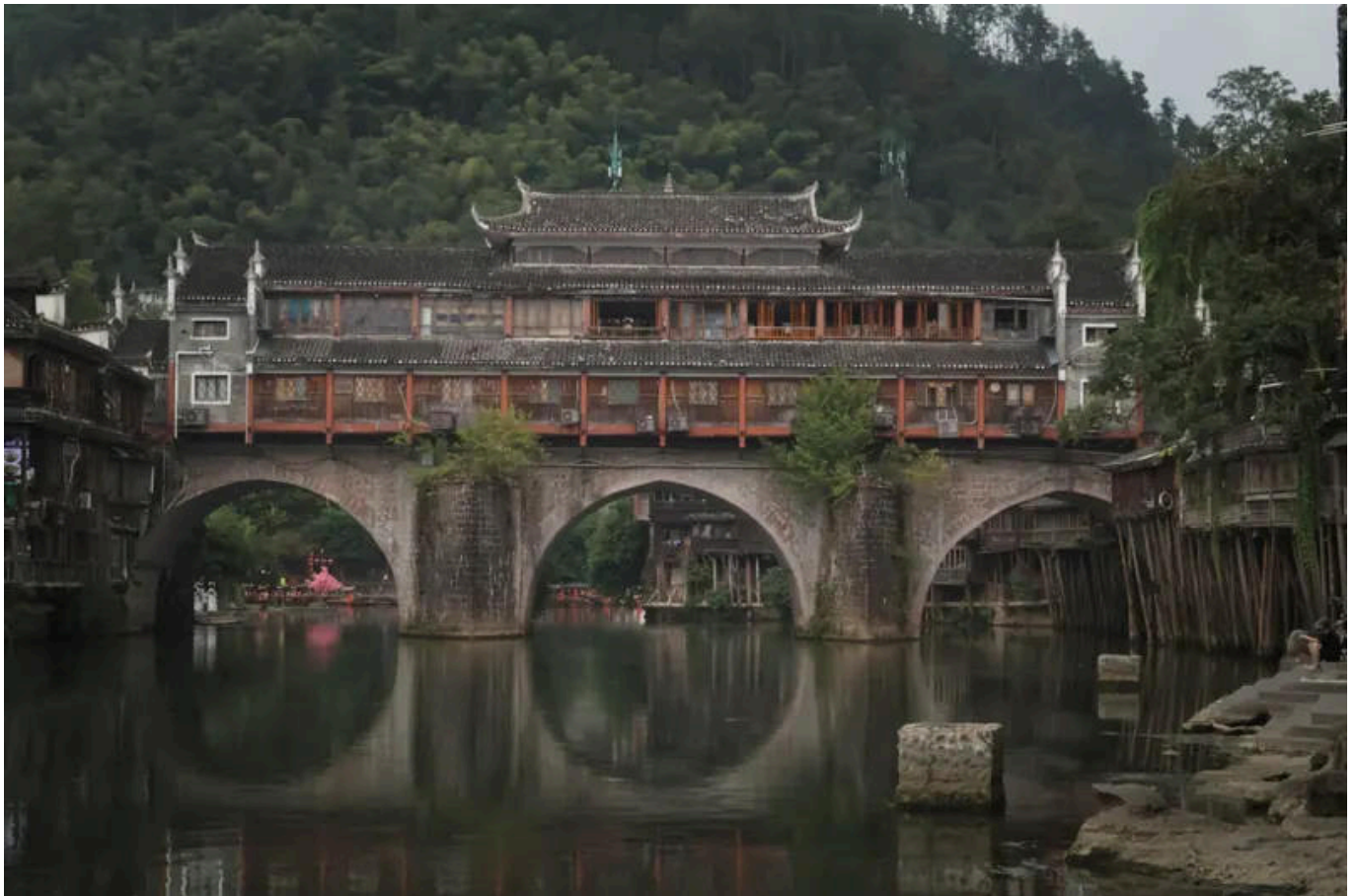
The covered bridge in Fenghuang.
